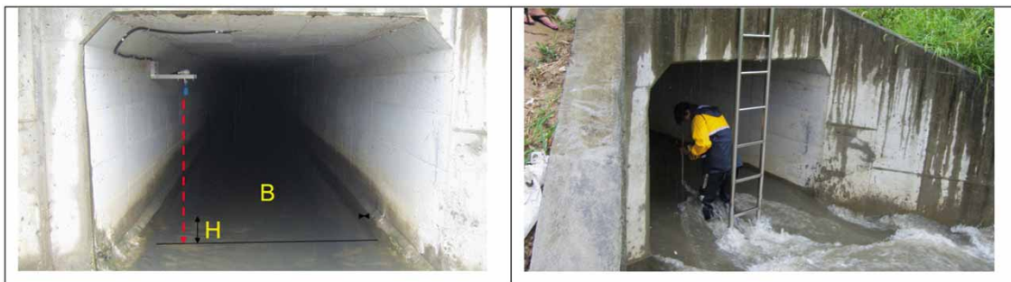
Figure 3 | Ultra sonic water level meter in storm sewer and field measurements for validation (Seo et al. 2009).
